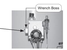
Step 8. Installation of Combination Thermostat/Gas Valve.
